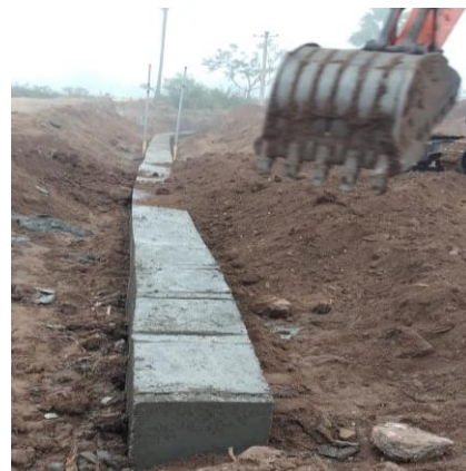
Sub-surface barrier under construction
