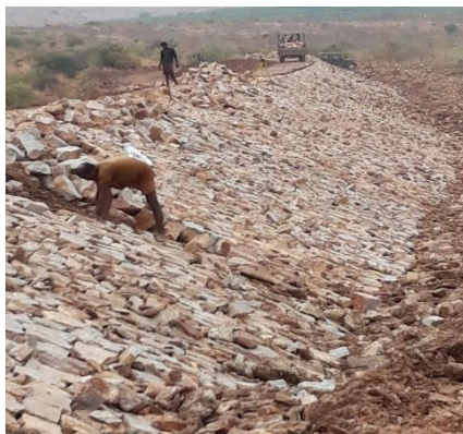
Percolation pond under construction
